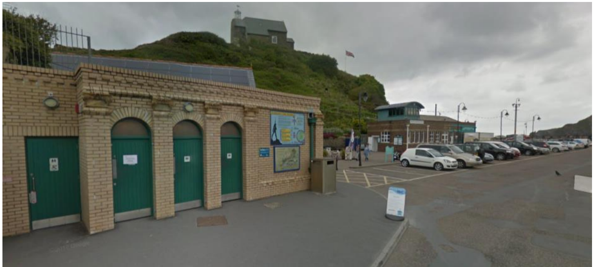
Photo of toilet block (accessible toilet is the first door on the left)
